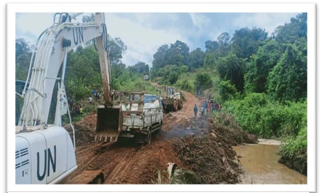
Engineering unit in MONUSCO supporting mobility
